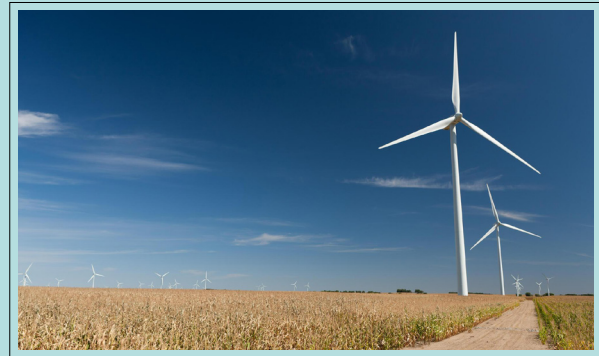
Energy sprawl is the largest driver of land use change in the United States, and TNC is offering science and tools to help site new development to avoid lands with high conservation values. © Richard Hamilton Smith
