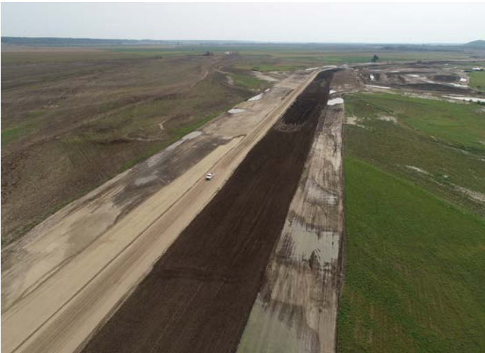
Levee composition work at L-536, September 2020.
