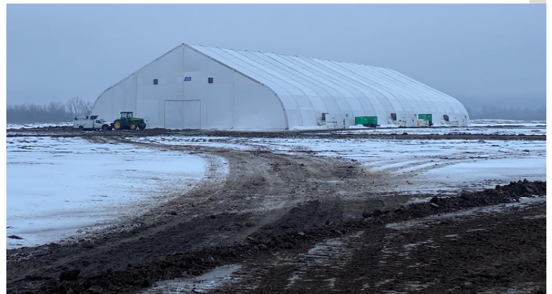
Warming tents were used to thaw the project's clay material during the last quarter of construction, Winter 2021.
