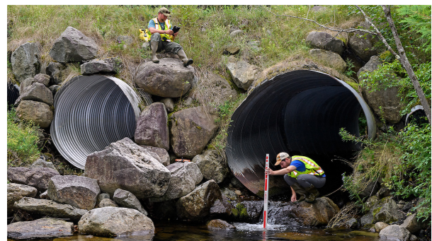
Culvert. © John DiGiacomo
