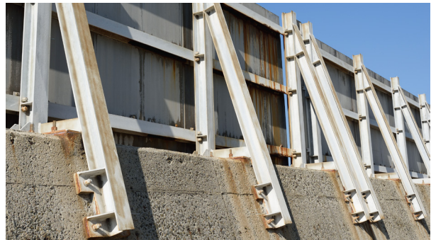
Concrete and steel breakwater seawall. © Akiyoko/iStock
