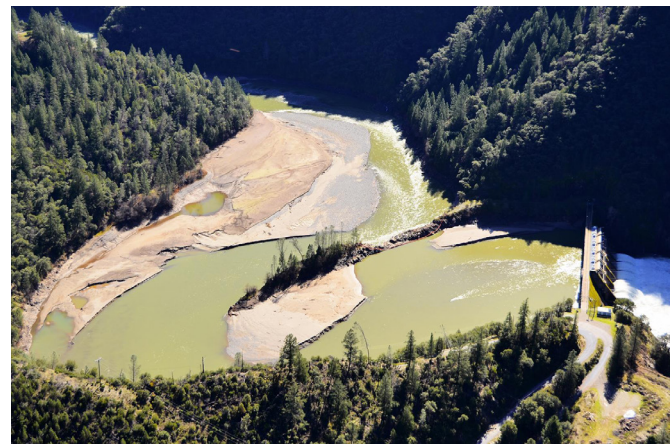
Sediment and debris build up near PCWA Ralston AfterBay Dam. © Placer County Water Agency
